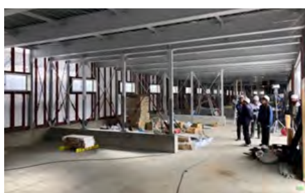
Building safety assessment
