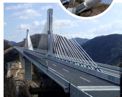
Shin-Meishin Expressway, Ikuno Bridge (NEXCO West Nippon)
