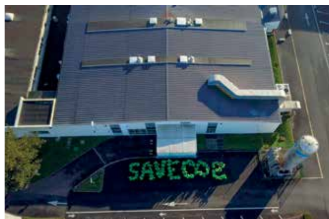
Schneider Electric’s Bourguebus site, France
