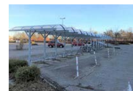
Parking lot at Böblingen
