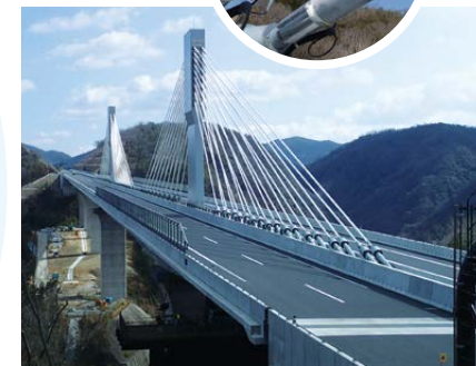
Shin-Meishin Expressway, Ikuno Bridge (NEXCO West Nippon)
