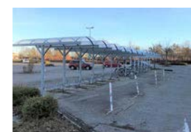
Parking lot at Böblingen
